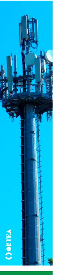
The acronym **BTS** stands for **Base Transceiver Station** and is used to indicate all the transmitting and receiving devices that enable the radio coverage in a telecom cell.
